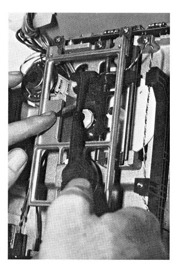
**FIG. 4–11** Changing the head load pad.
