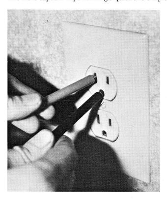
**FIG. 6–2** Checking an outlet with a meter.
